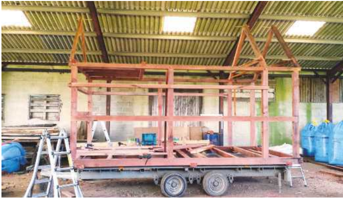
The basic frame is constructed on its trailer
